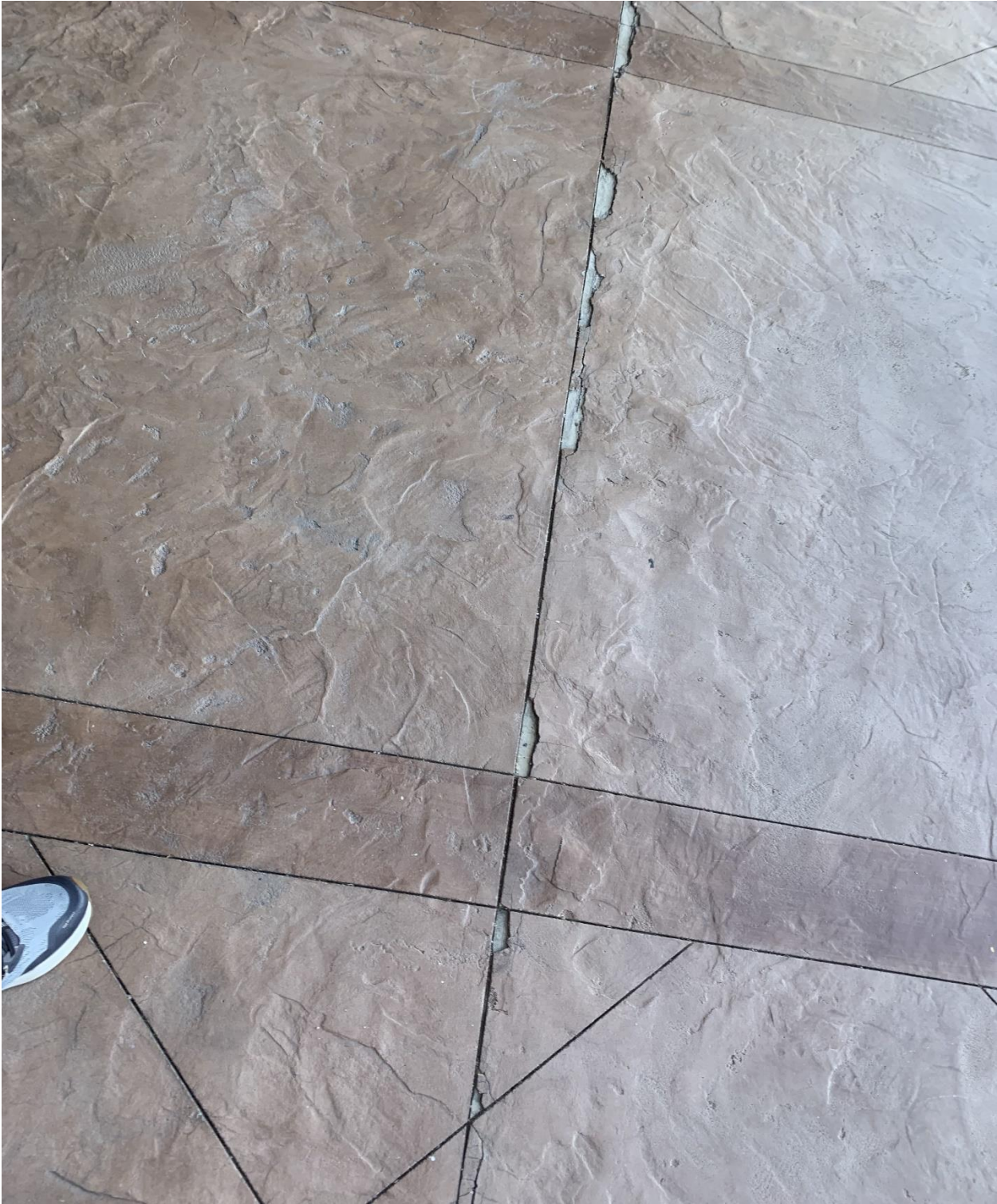
Patch/match concrete at entrance
