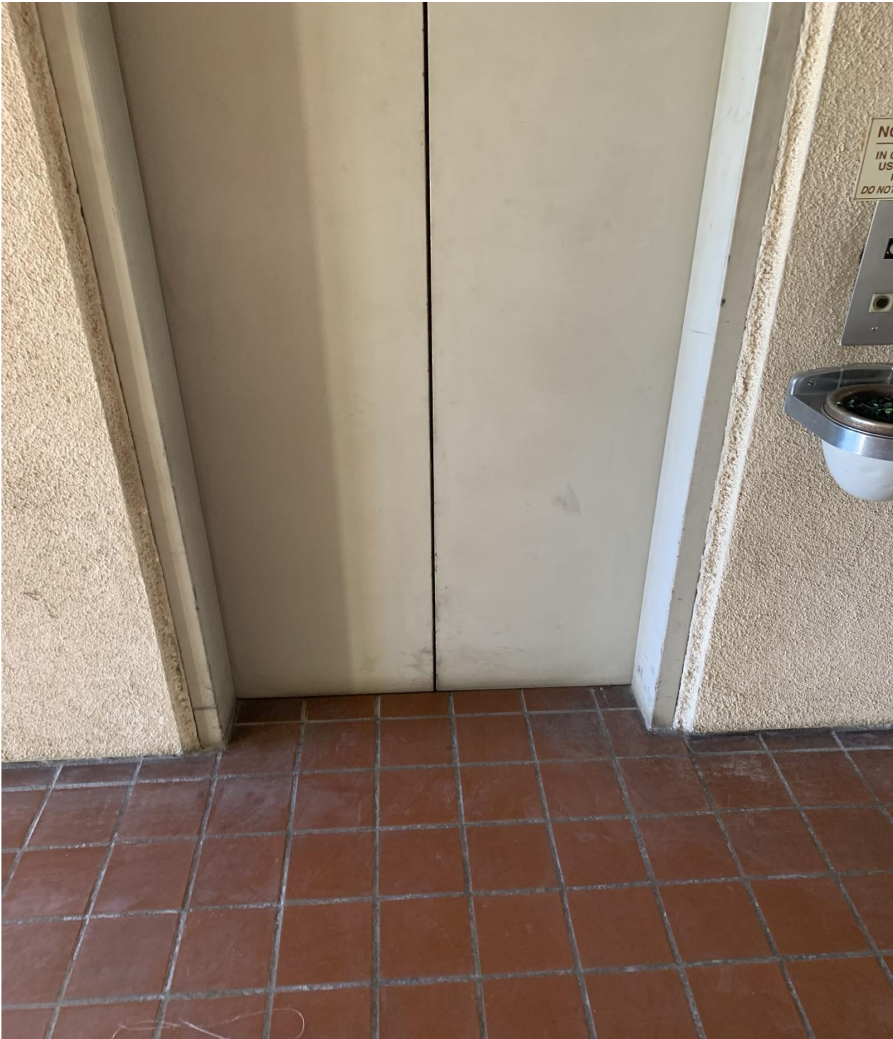
Paint elevator door 1 st floor east
