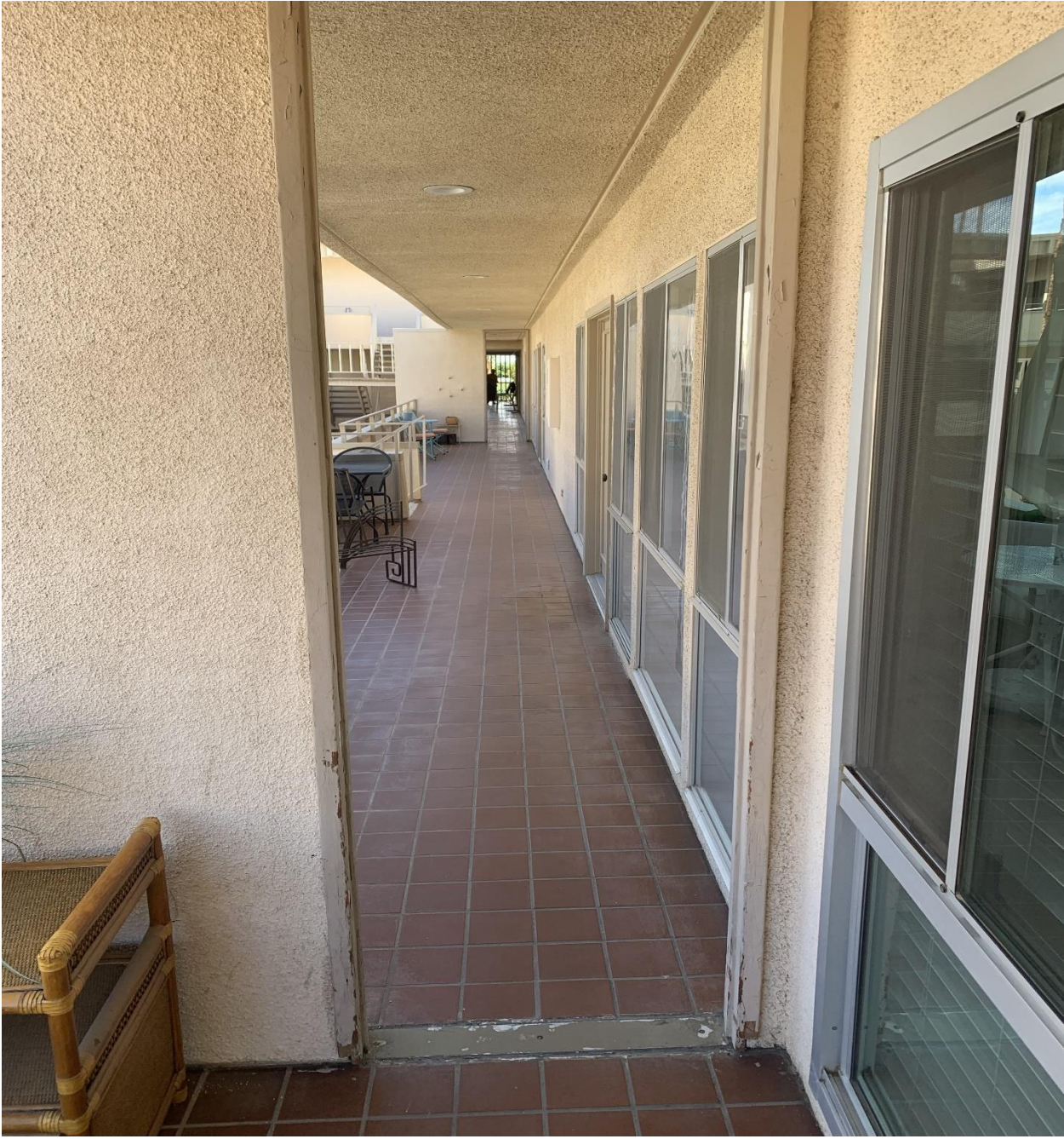
Paint pass-thru between 222 and 221
