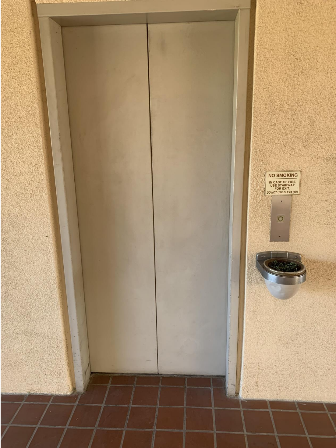
Paint 3 rd floor northwest stairway door and elevator
